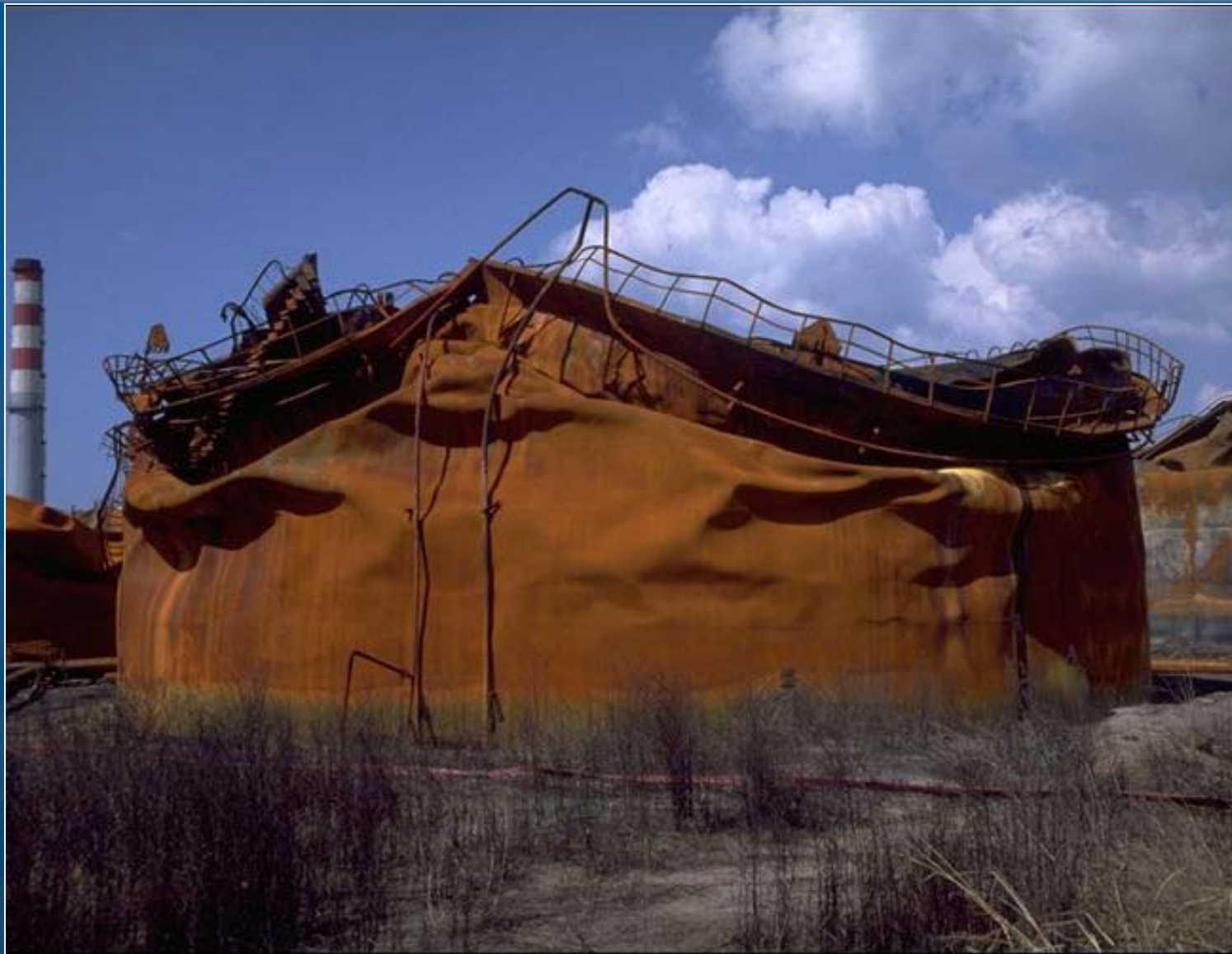
Situation of tanks after fire
