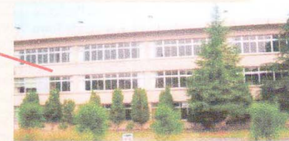
Before retrofit (outside view)
