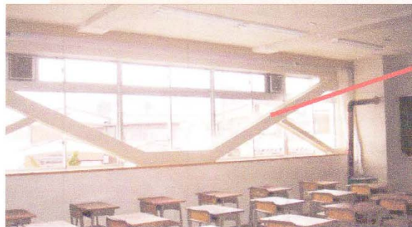
After retrofit (Inside view)
