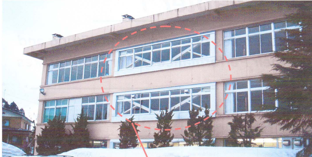
After retrofit (outside view)
